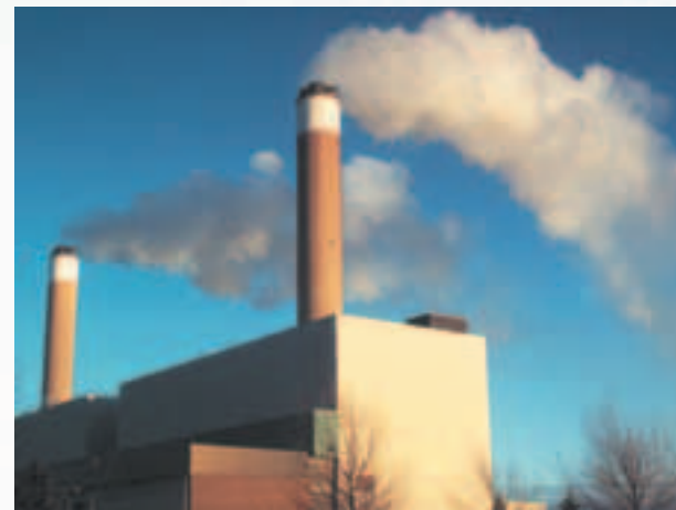
THE NANTICOKE GENERATING STATION LOCATED ON LAKE ERIE, ONTARIO, HAS BEEN CALLED 'THE SUV OF POWER PLANTS.' IT IS CANADA'S BIGGEST SINGLE SOURCE OF AIR POLLUTION.
